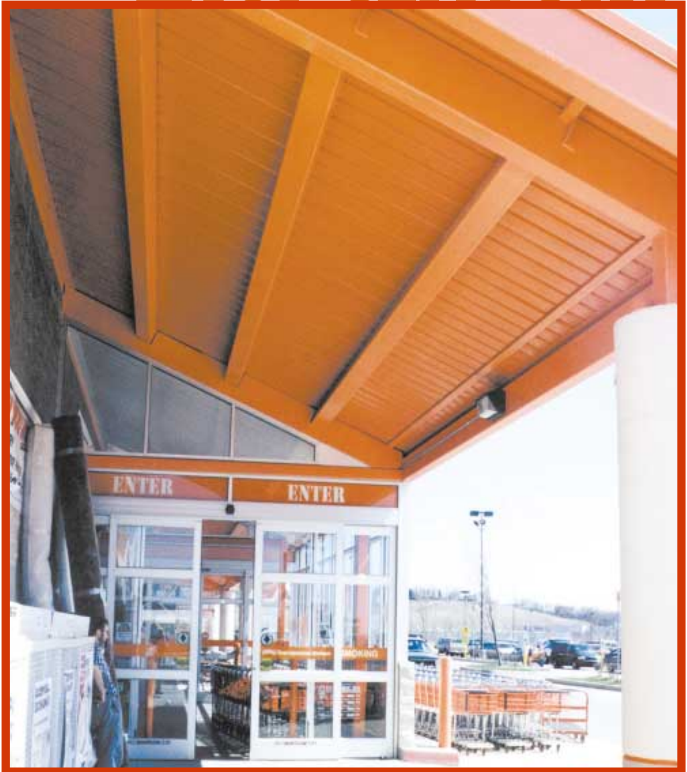
Columns and Canopy Supports for Home Depot Stores
