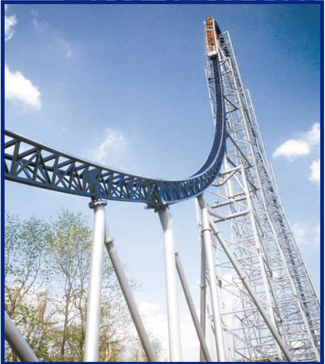
Cedar Point's new Millennium Force coaster uses 5,000 tons of HSS.
