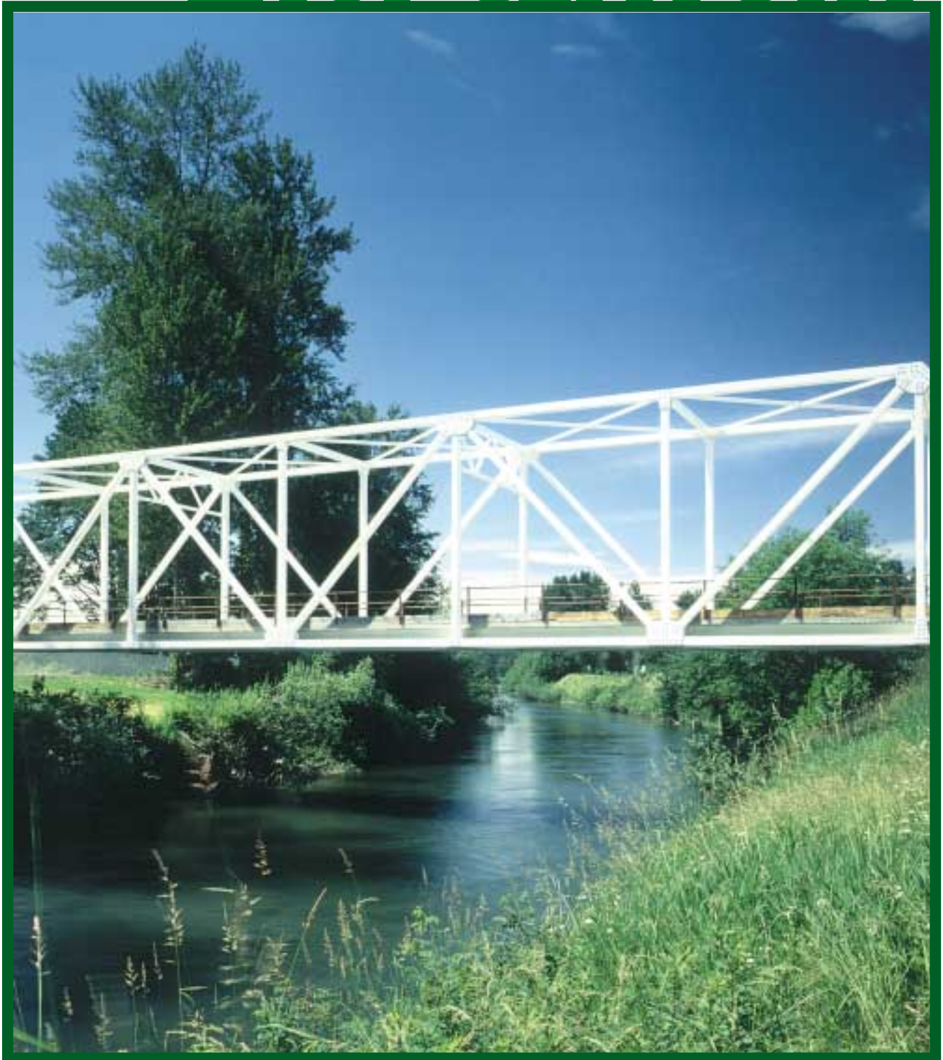
Green River Trailway Bridge, Kent, Washington
