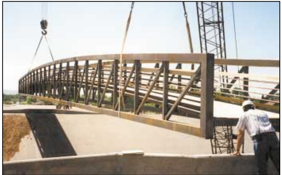
Installation of modified bow bridge, Albuquerque, New Mexico
