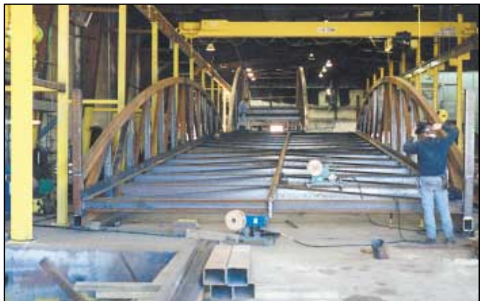
Bridge fabrication at Steadfast's Fort Payne, Alabama plant
