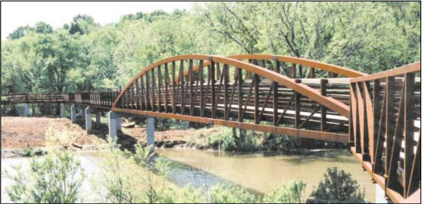
Bow truss bridge, Murphreesboro, Tennessee
