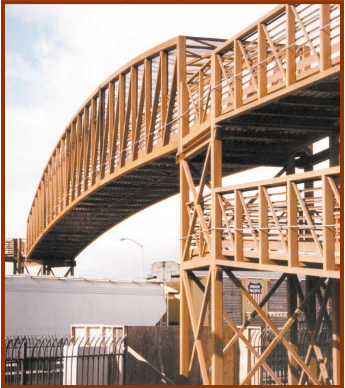
This 158-foot-long pedestrian railroad overpass with ramps in San Luis Obispo, California, typifies the use of HSS in spans built by Steadfast Bridges.
