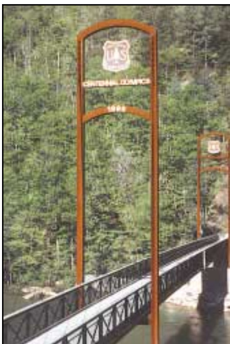
Cable-stayed pedestrian bridge, Ocoee, Tennessee
